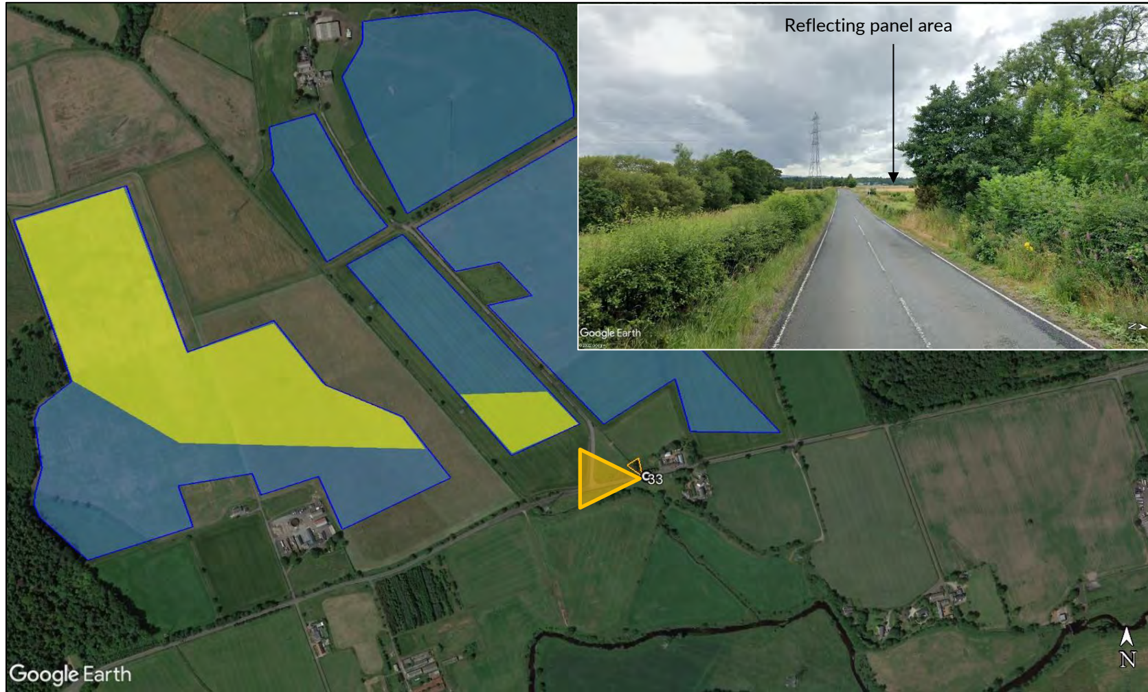
Figure 18 Point-of-view from road receptor 33
