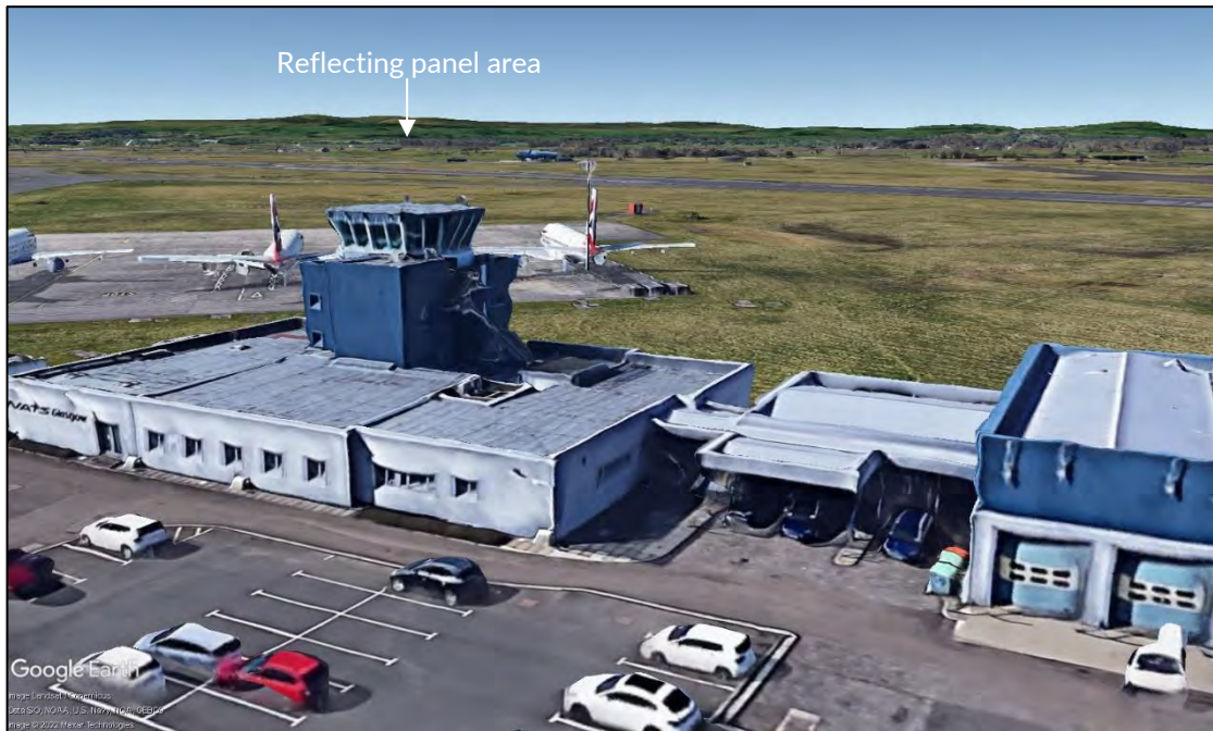
Figure 11 Viewpoint of reflecting panel area from ATC Tower
