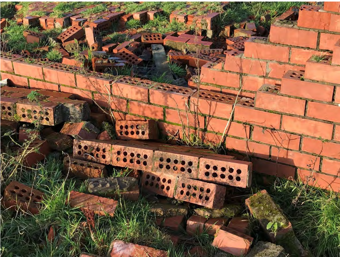
Plate 4: Detail of building showing 21st-century brickwork
