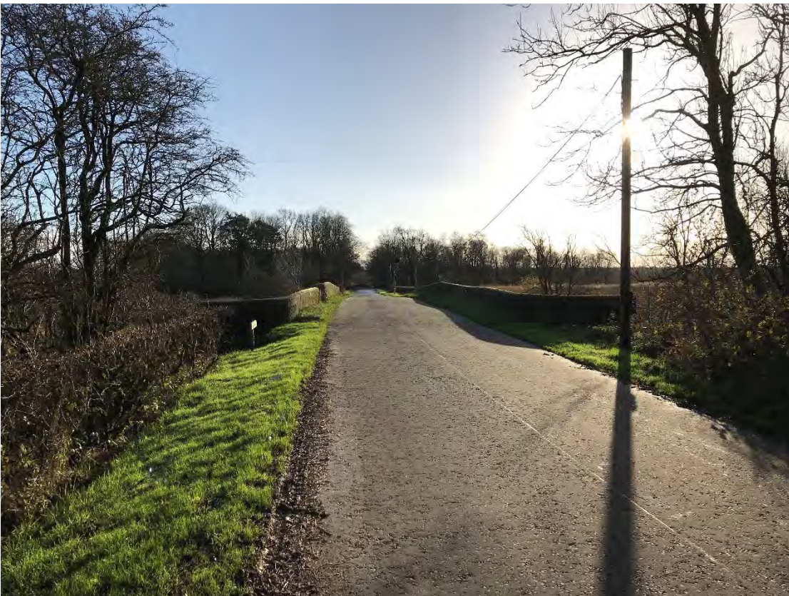
Plate 17: Fulwood Bridge seen from the north
