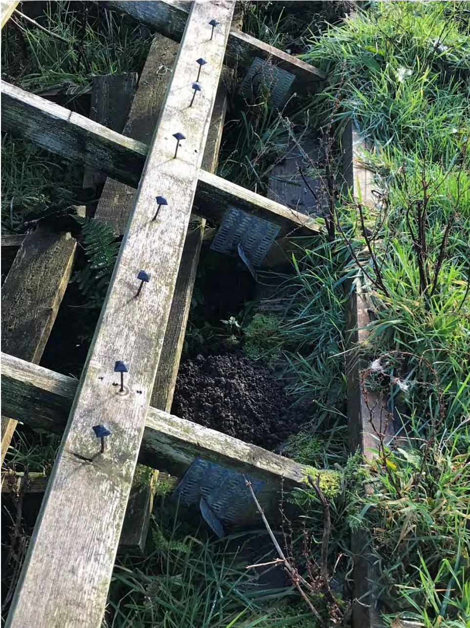
Plate 5: Detail of roof showing fasteners
